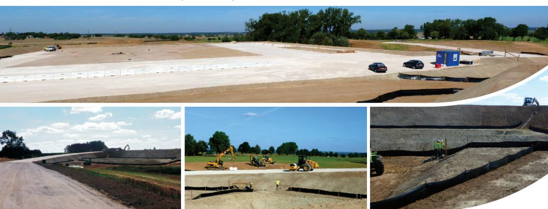
The drill site and its access road of 10 m width and 273 m length was reinforced with crushed-stone aggregate 0-63 of total 8200 tons and mechanically stabilized non-swelling soil of total 18000 tons. Total earthworks balance - 24000  $m^3$ . The site's surface was additionally reinforced with composite sheets of total 4475  $m^2$ . Works completion time - 6 weeks.
