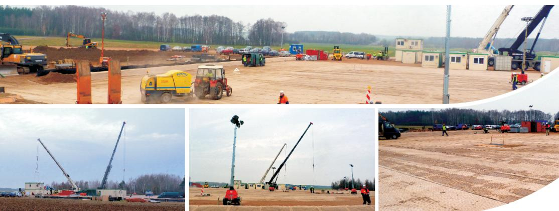
The drill site and its access road of 10 m width and 125 m length was reinforced with crushed-stone aggregate 0-31,5 of total 9500 tons and mechanically stabilized sand and gravel mix of total 17300 tons. Total earthworks balance - 21500 m³. The site's surface was additionally reinforced with composite sheets of total 4475 m². Works completion time during autumn-winter period - 5 weeks.
